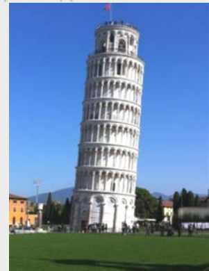
The micro-piling technology saved the historical Leaning Tower of Pisa.
